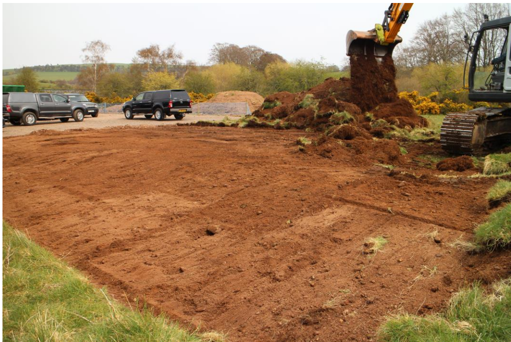
Plate 6: Stripping of the topsoil (06/05/16) prior to extending the car parking area at the south west side of the site (at c NGR 355665 645380) facing north-eastwards
