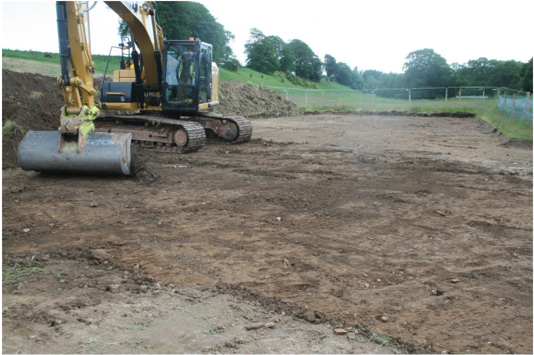
Plate 9: Topsoil stripping of an area (45m x 70m) adjacent to the escarpment on the eastern side (at c NGR 355833 645330) facing south-south-west
