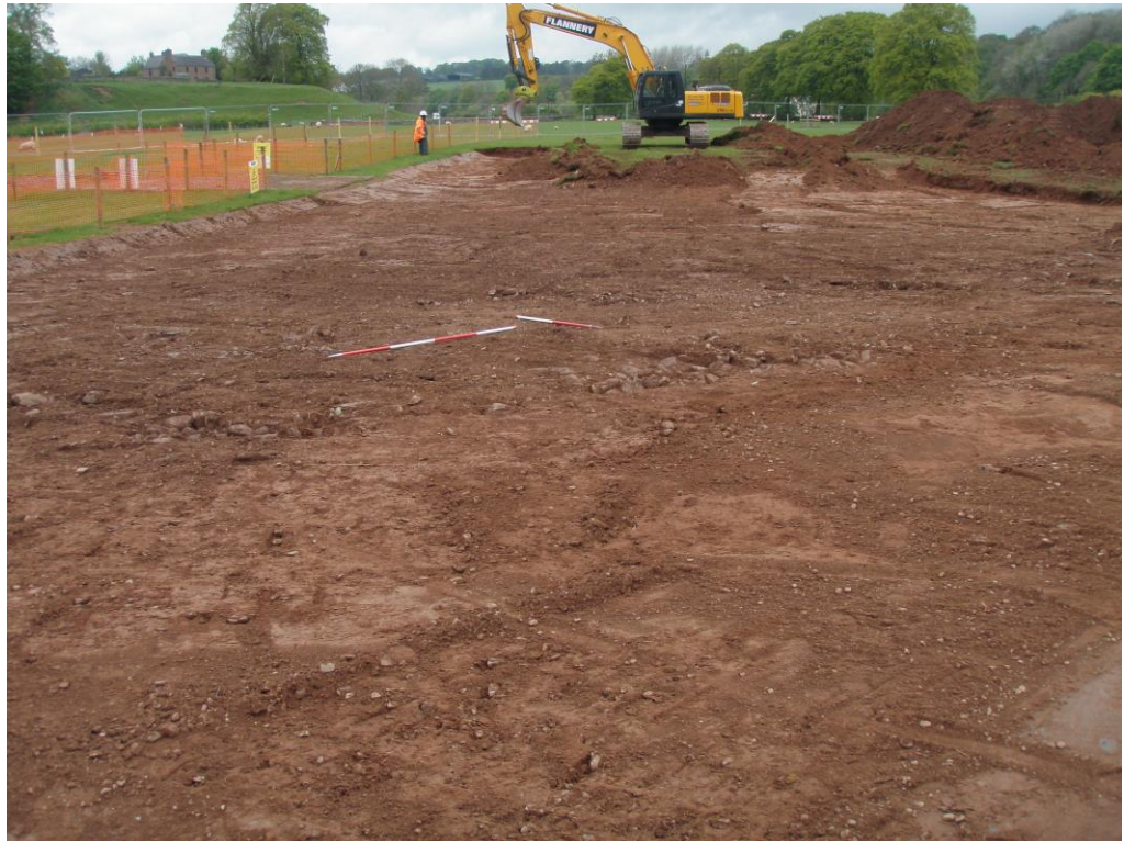
Plate 2: Topsoil stripping on the west side of Leader Water to the north of the existing gas pipe facing north-west (at c NGR 35700 64565). Layer 002 is visible across much of the area and the underlying deposit, 003 , comprises the large stones in the middle of the image
