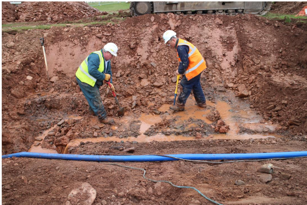
Plate 4: Excavations on the west side of the site (at c NGR 355694 645531) to reveal the existing gas pipe (600NB No 10 FEEDER) facing north-north-east
